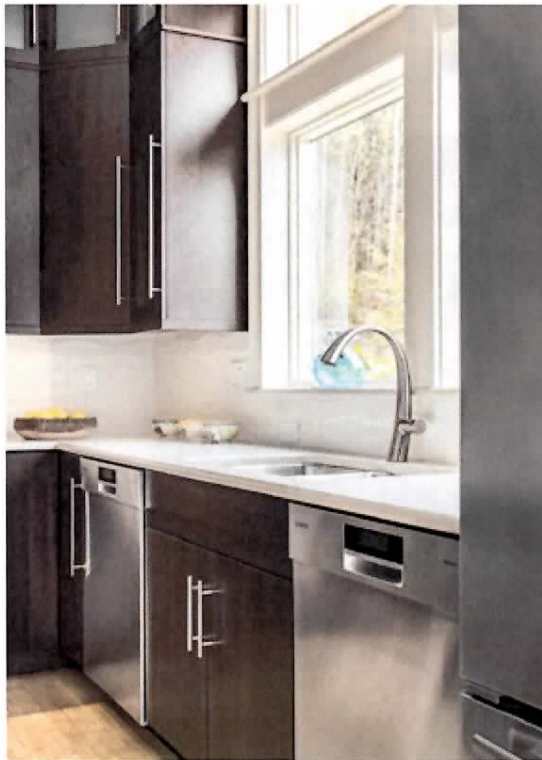
Top: To gain more storage, the cabinets were extended all the way to the ceiling. The clerestory cabinets repeat the design of the window, which was moved from the corner to the side wall to make the space more efficient.
